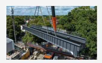
Roßlauer Schiffswerft carried out dismantling and assembly work at the Wandsbek-Gartenstadt subway station in Hamburg. Two old steel bridges were excavated and a new steel trough bridge was lifted into place.
